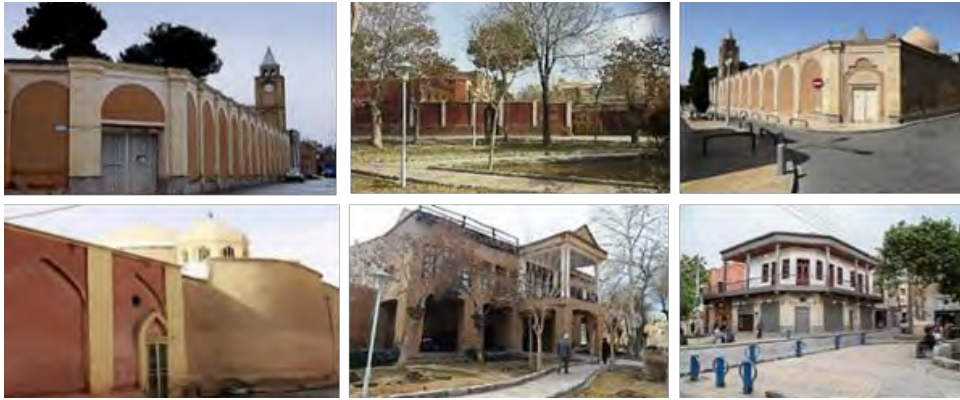
Fig.4. Buildings with architectural value in the Jolfa neighborhood
