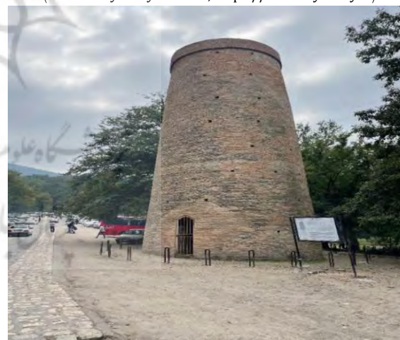
Fig. 4: Water pressure relief tower, By Authors
