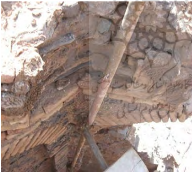
Figure 7: Overhead view of the decorations – collapsed ceiling
