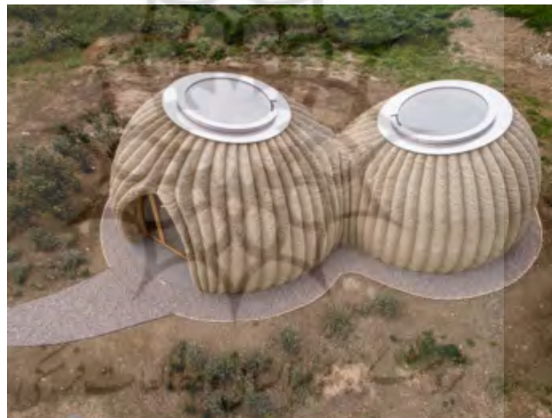
Fig 7: Tekla project built with native materials and self-standing roof form by wasp (Moretti, 2023)
