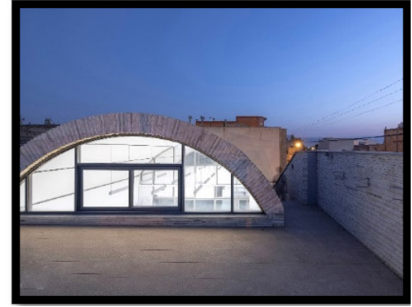
Fig.6 - Tak-Taagh house in Najafabad (Source: CAOI Website)
