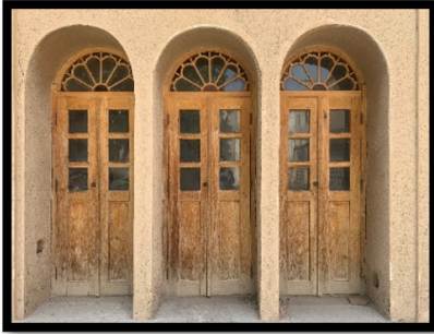
Fig.4 - Kahkeshan house in Isfahan (Source: Researcher)
