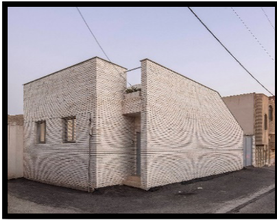
Fig.1 - Tak-Taagh house in Najafabad (Source: CAOI Website)
