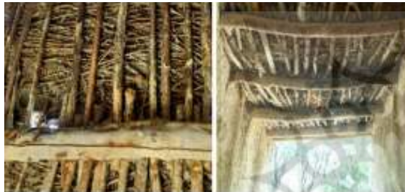
Fig. 11. Details of the roof of the Kech
