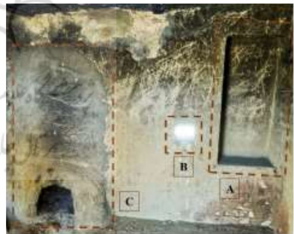
Fig. 10. Internal elements of the Kech: A. Ledge. B. Olune. C. Fireplace
