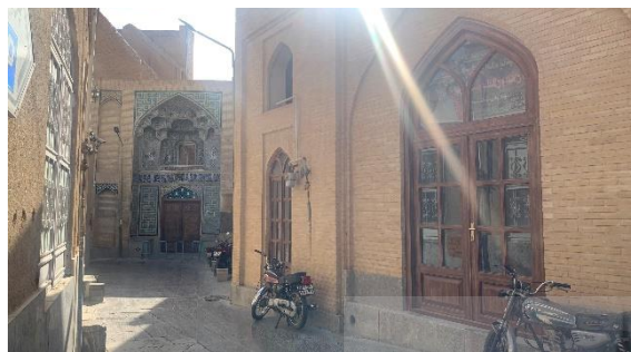
Fig. 18. A view of rooms that located on the north side of Hakim Mosque
