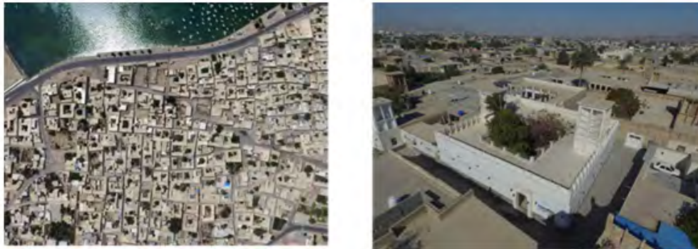
Fig. 1: (a)The historical context of Bandar-Kong (b)windcatchers in Bandar-Kong
